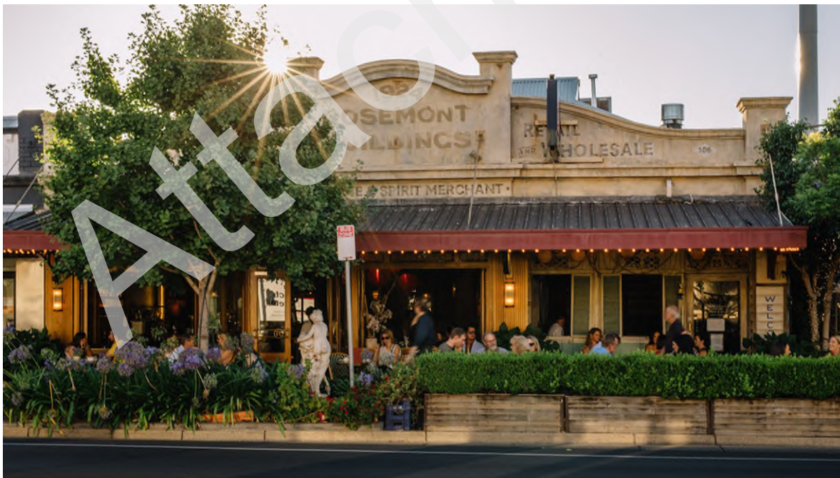
Original Rosemont Buildings, currently being reconstructed https://glamadelaide.com.au/re-build-begins-at-rosemont-hall-after-devastating-fire/
