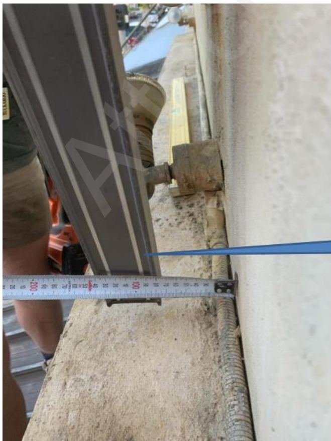
Photo 2 – Photo provided by make-safe contractor showing wall displacement from vertical spirit level
