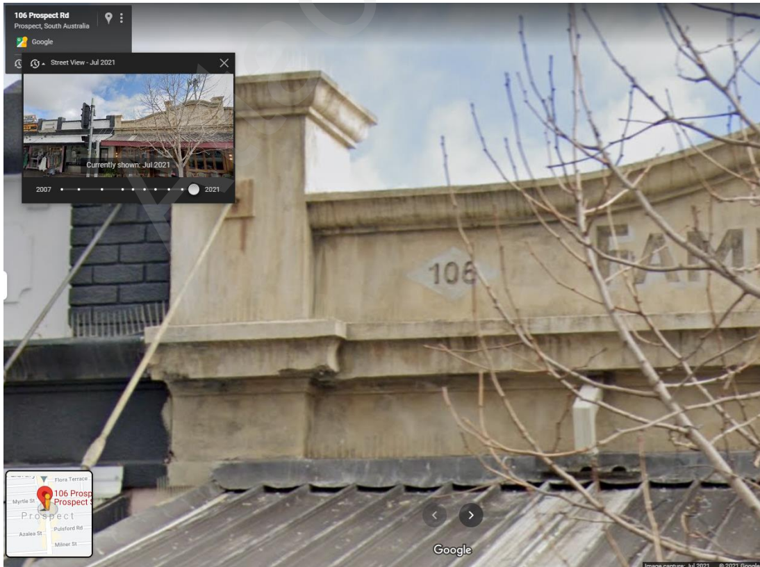
Photo 4 – Google Street View image dated July 2021
