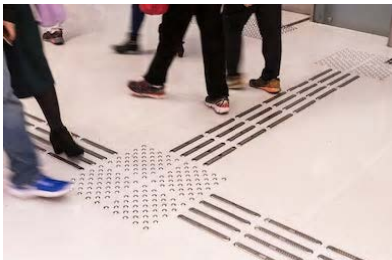
Figure 3. Examples of tactile and directional paving.
